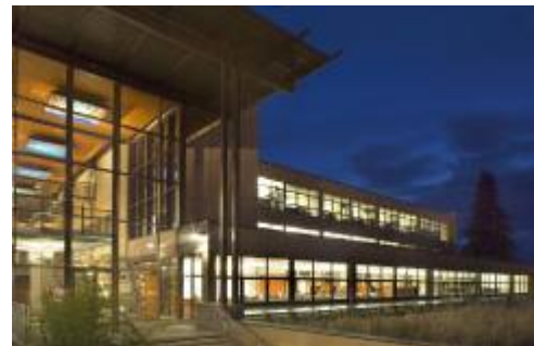
County Administration Building, 2015
