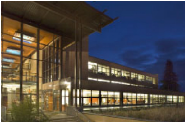
Kitsap County Administration Building www.wbdg.org
