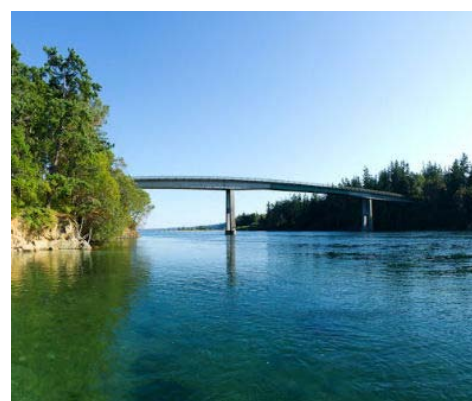
Figure 4.4.8. The Portage Canal Bridge connects the Olympic Peninsula and Indian Island (photo credit: NWicon).
