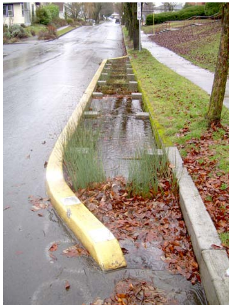
Figure 4.5.5. Example of green stormwater infrastructure emulating natural drainage, where carefully chosen plants and soils treat stormwater runoff and allow infiltration to reduce water pollution.
